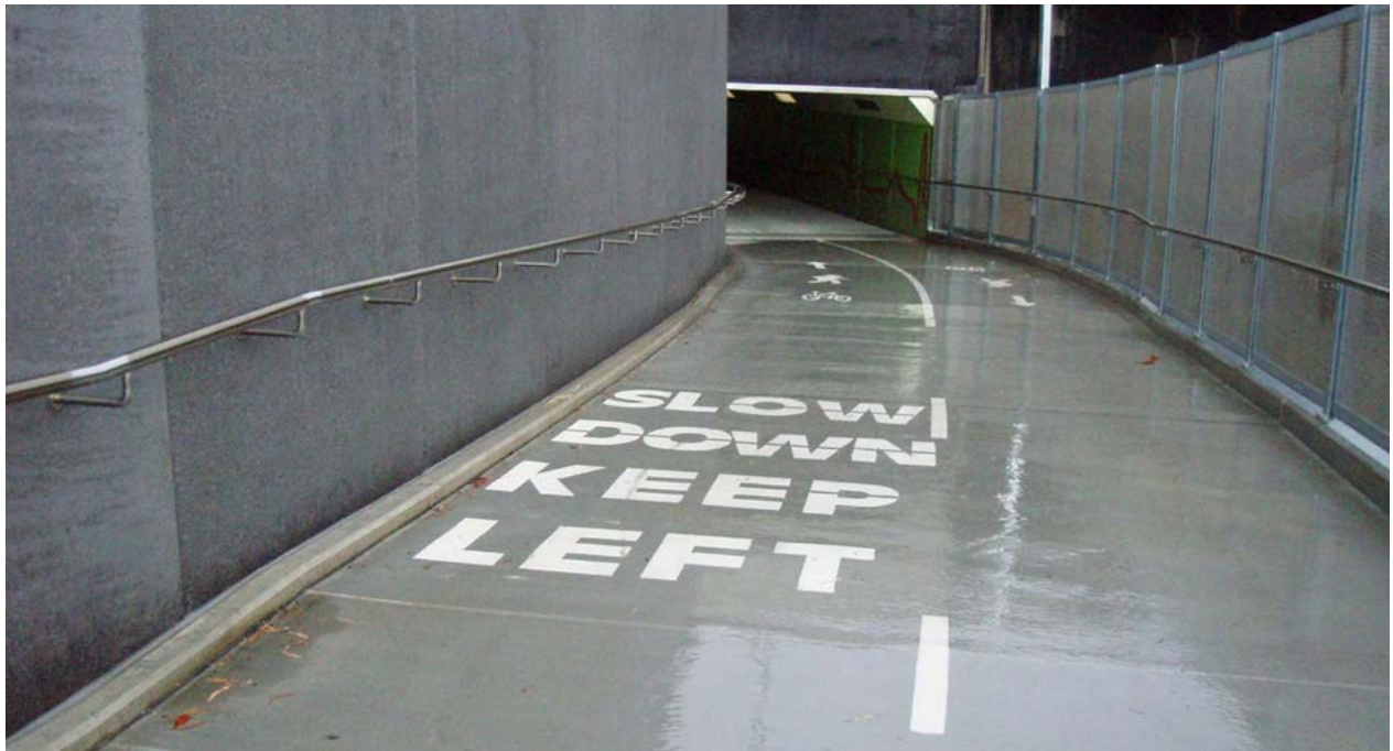
Figure 9: Pavement markings use on a sight restricted corner to manage approach speed
