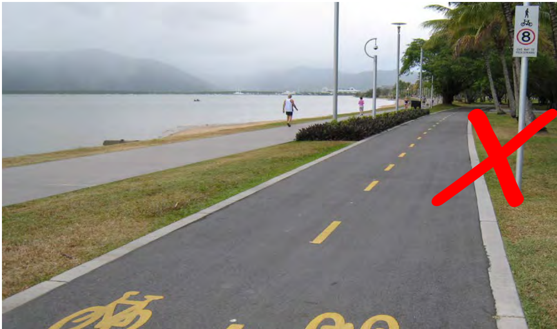
Figure 2: Inappropriate speed limit signage application
