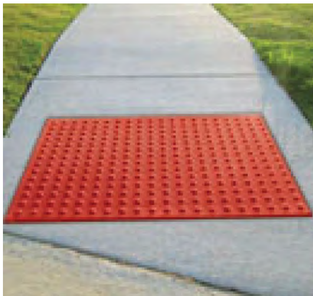
Figure 6-7 Example Image of Detectable Warning Surfaces
