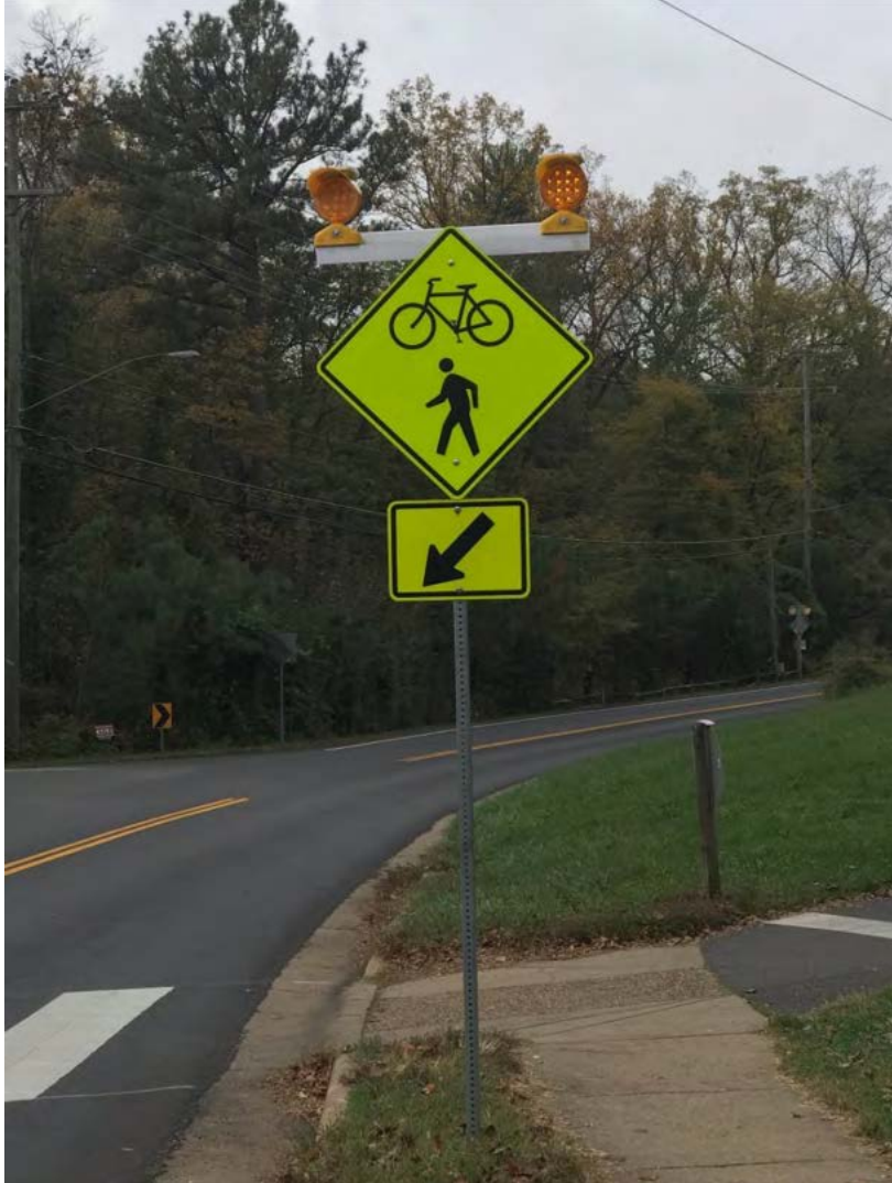
Figure 6-1 Temporary Flashing Beacon at Shreve Road W&OD Trail Crossing
