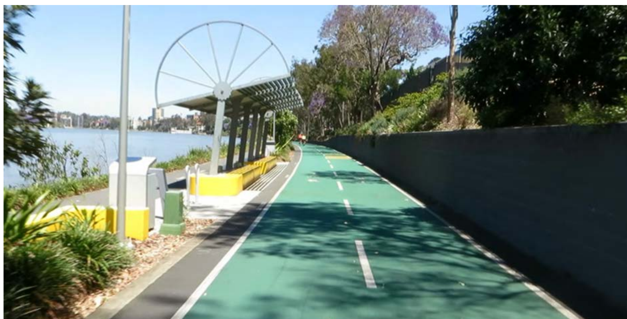
Figure 6: Use of segregation and pavement markings to minimise conflict
