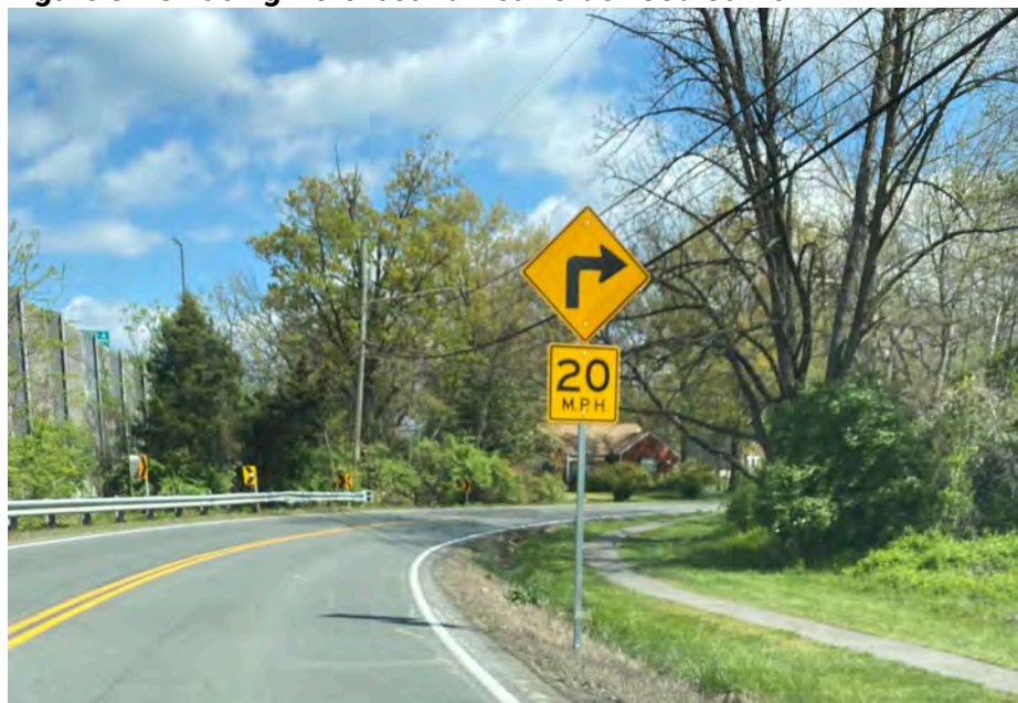
Figure 3-23 Facing Northbound Near Oldewood Curve
