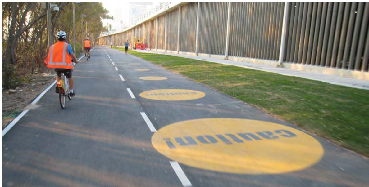
Figure 3: Effective use of pavement markings to manage speeds
